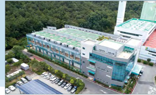
Busan Green Energy (30 MW)
